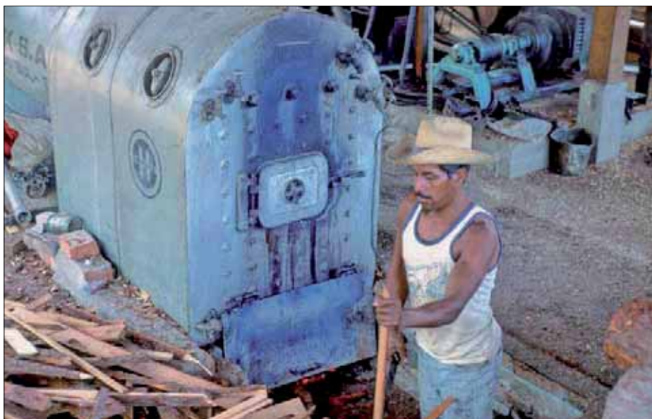
The cost of electricity generated from woodfuels depends on a wide range of factors, including the cost of feedstock and the technology employed; here, wood scraps fuel a boiler for electricity production in Honduras
